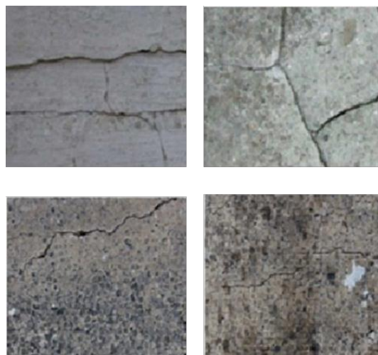
Figure 1. Top row shows high contrast, low clutter images, Bottom row shows real surface cracks
