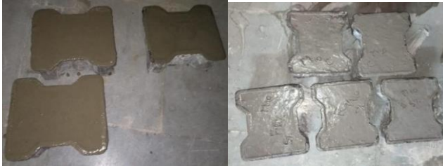
Fig.2 Concrete casting of interlock
